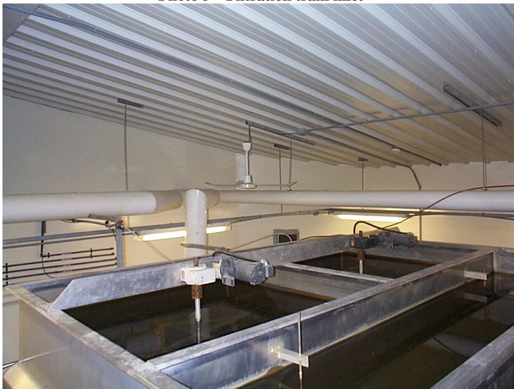
Photo 6 – Filtration train – Flocculation tanks
