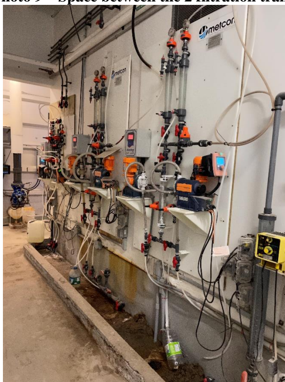
Photo 10 – Chemical dosing pumps
