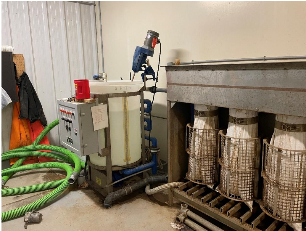
Photo 13 – Dewatering bagger system
