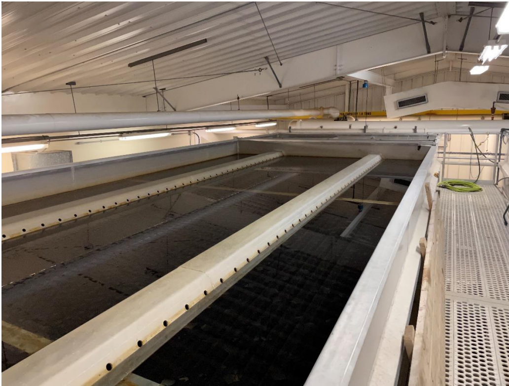
Photo 7 – Filtration train – Clarifier
